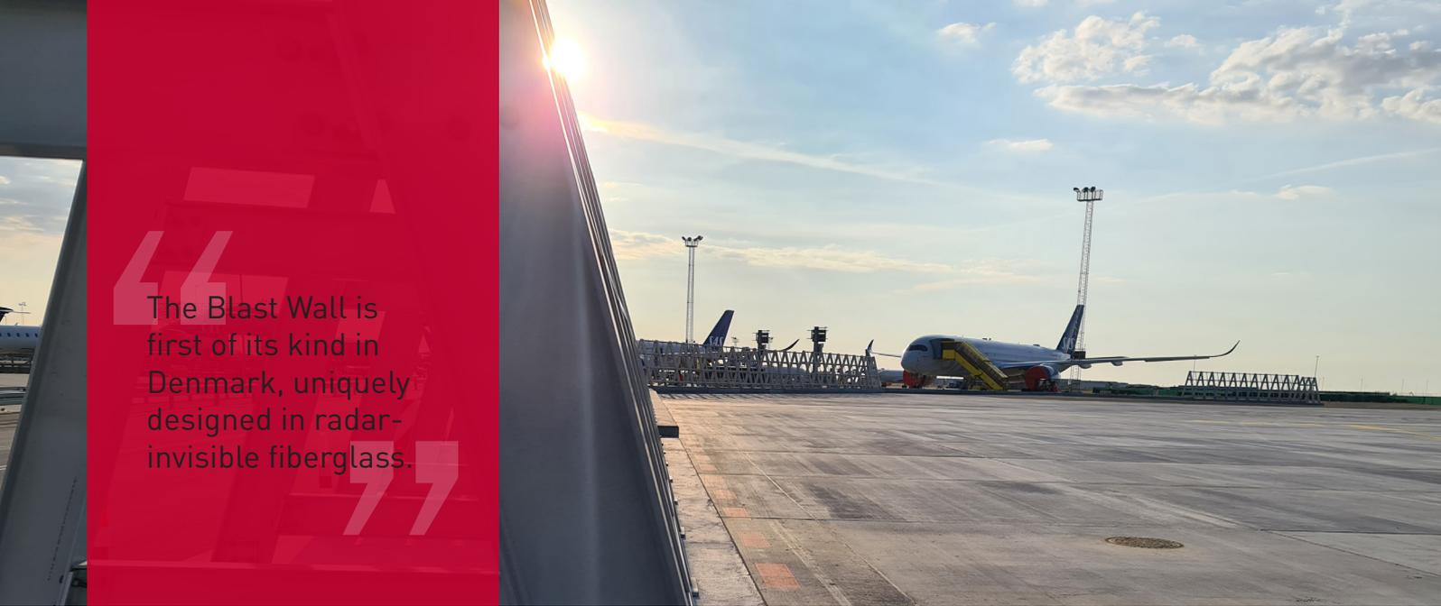
The Blast Wall is first of its kind in Denmark, uniquely designed in radar-invisible fiberglass.
